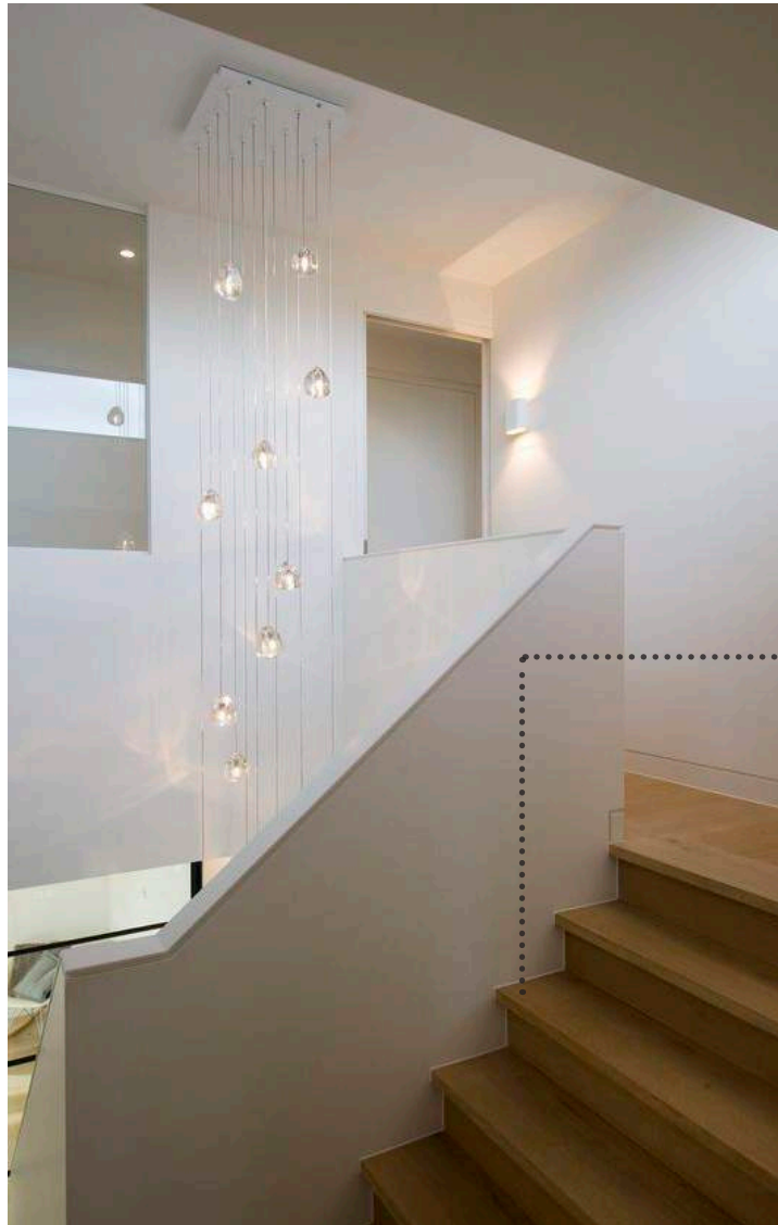
CLOSED TREAD AND DRYWALL RAILING TO START AT LANDING AND CONTINUE UNTIL 2ND LEVEL
